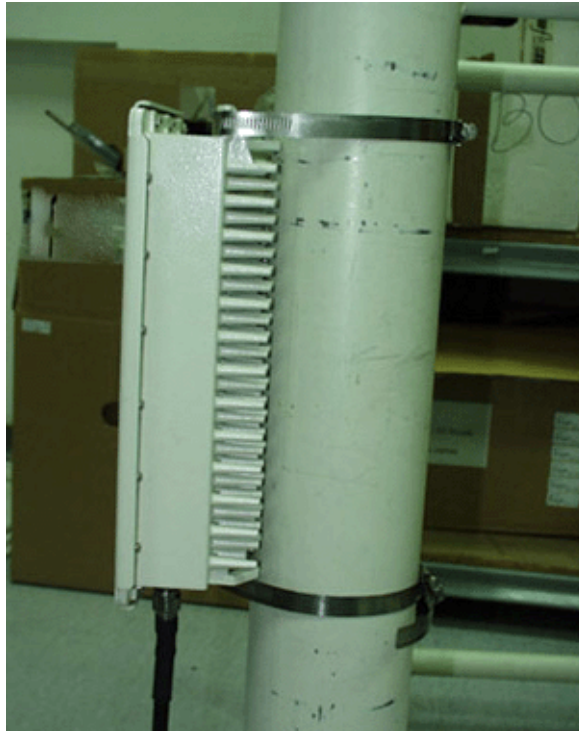
Figure 5-27: Securing the AU-ODU to the Pole - 3
