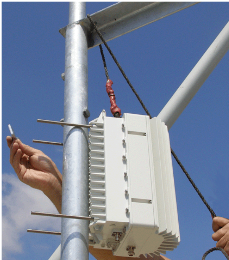
Figure 5-20: Lifting the AU-ODU Using a Harness - 2
